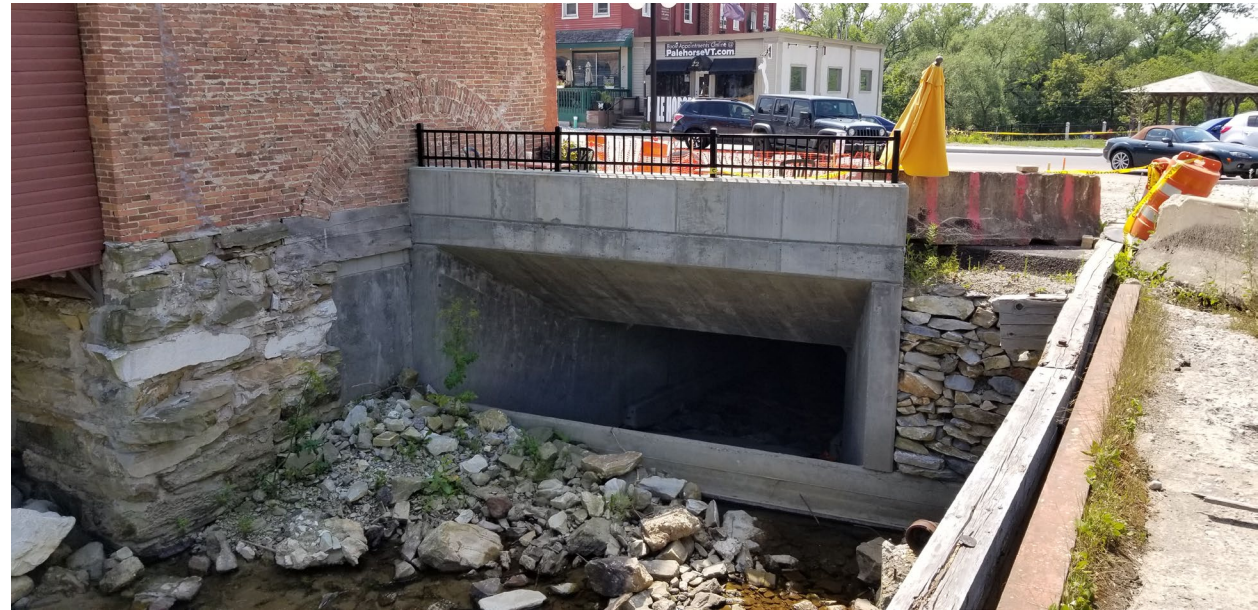
Center Street Overflow Culvert
