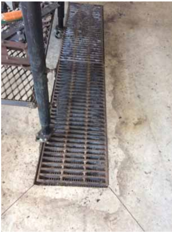
Floor trench drain
