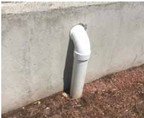
Figure 12: Unsealed exterior wall penetration(s).
