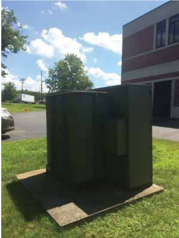
Figure 5: Exterior pad mount transformer.
