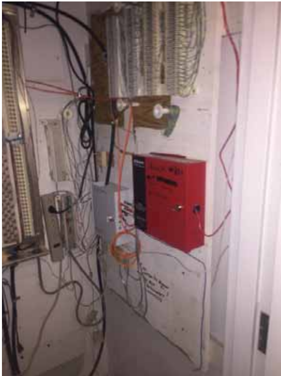
Figure 7: Telcom / Security Panels (Source: MSK)
