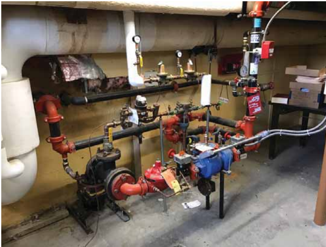
Figure 25: Basement sprinkler riser
