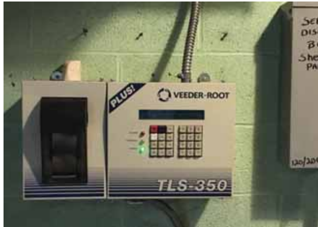
Figure 11: Emergency Generator Tank Monitor
