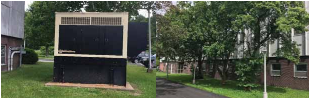
Figure 15: Pad mounted Generator (SE corner)
