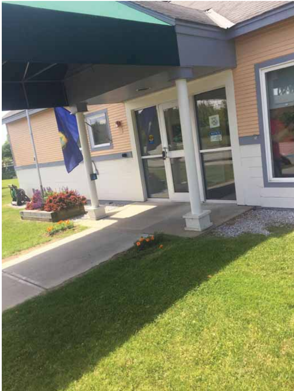
Figure 1: Front Entrance looking Southwest (photo credit: MSK Engineering, Inc.)
