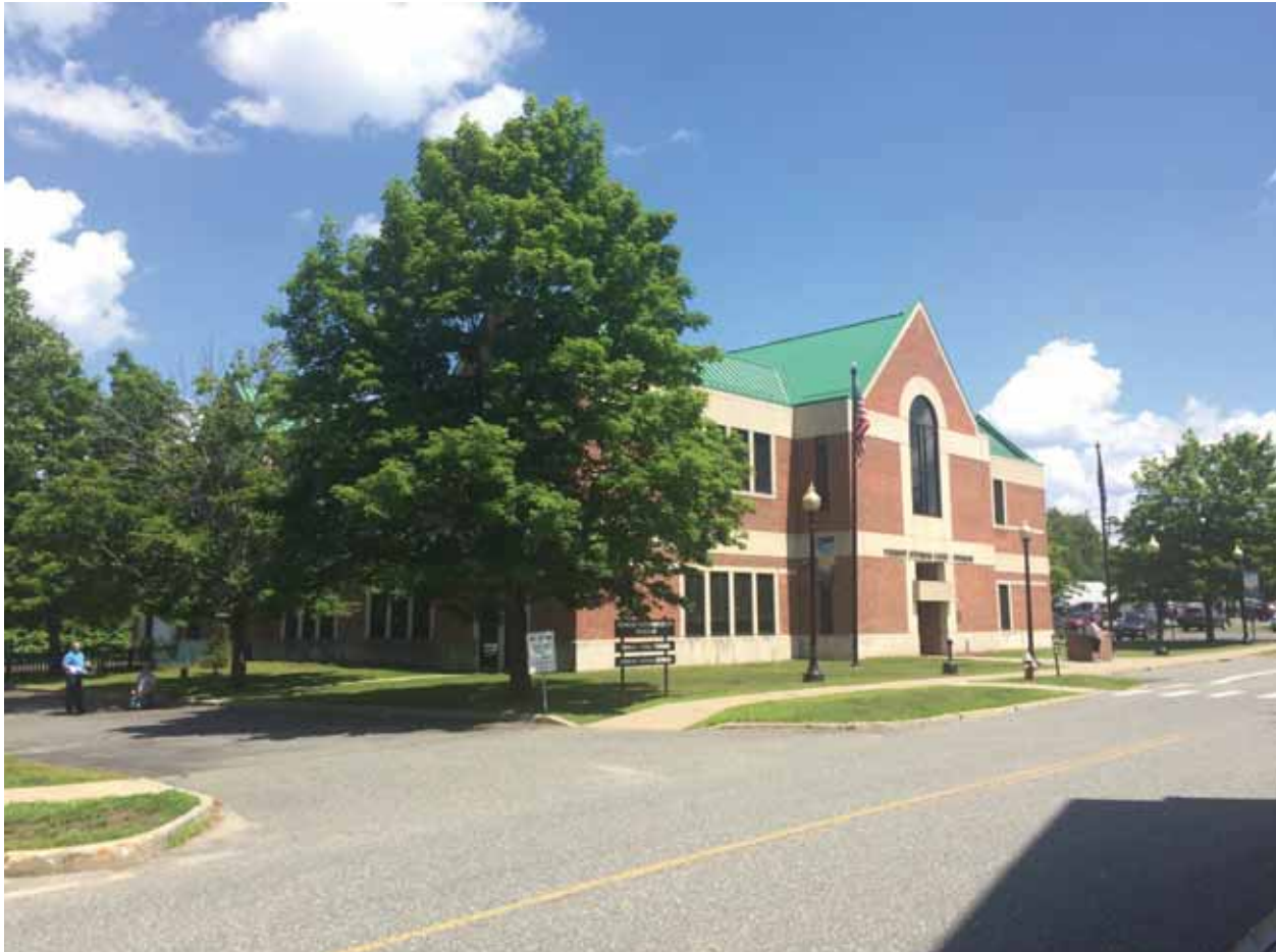
Figure 1: Front entrance looking east (photo credit: Freeman French Freeman)
