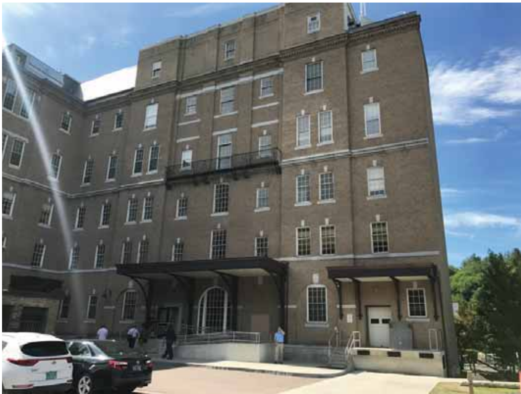
Figure 6: North façade and rear entrance
