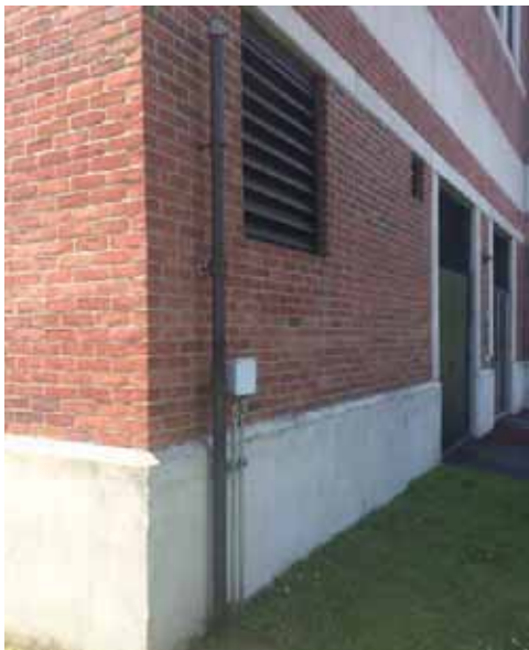
Figure 7: Vent pipe (underground fuel tank?).
