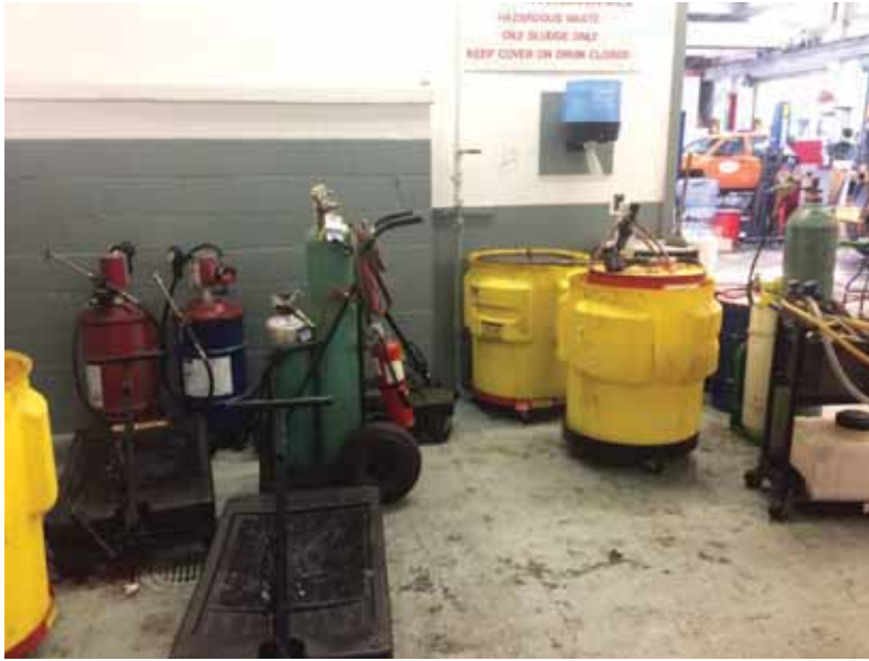
Contents could be hazardous if not addressed prior to flood event
