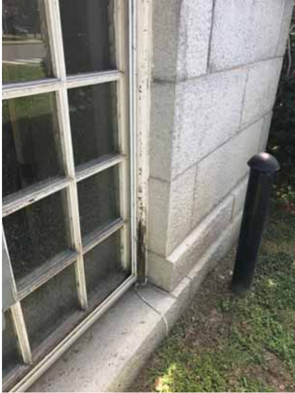
Figure 27: Basement window (typical)
