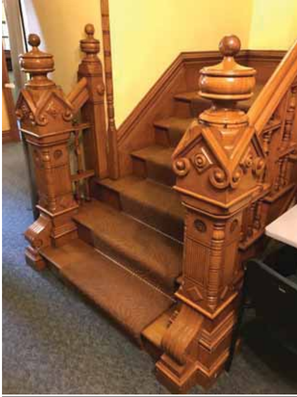
Figure 16: First floor woodwork (understood to be above predicted flood elevations)
