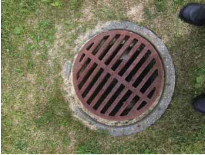
Figure 11: Exterior drainage structure
