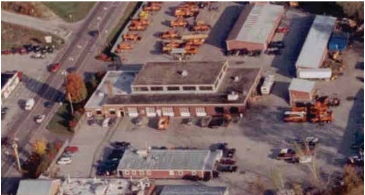
Figure 2: Historic overhead view of Central Garage Building (photo credit: VTrans)
