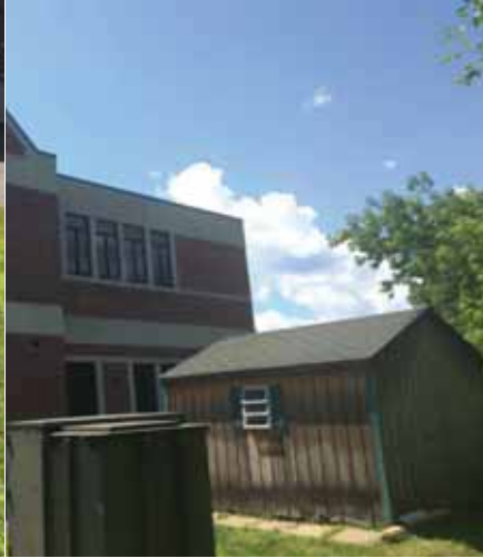
Figure 6: Exterior Storage Shed.
