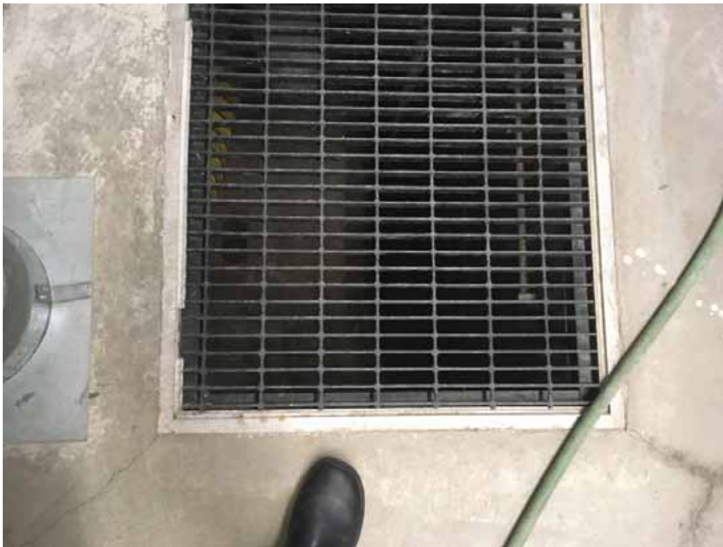
Figure 12: Sub-basement floor access grate to lower areaway(s)
