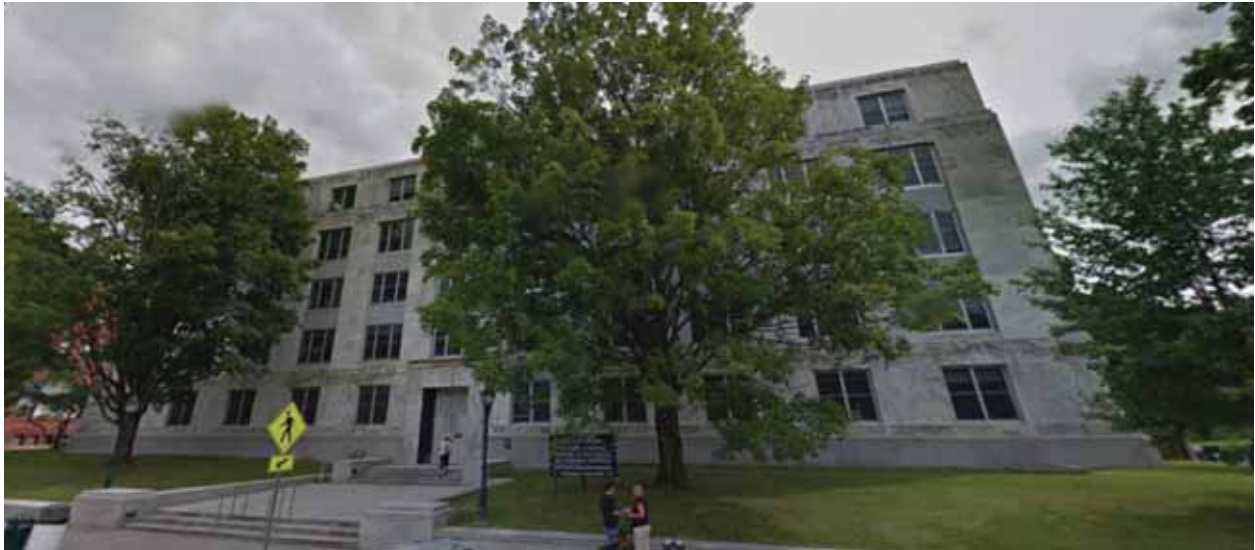
Figure 2: North Façade (photo credit: Freeman French Freeman)
