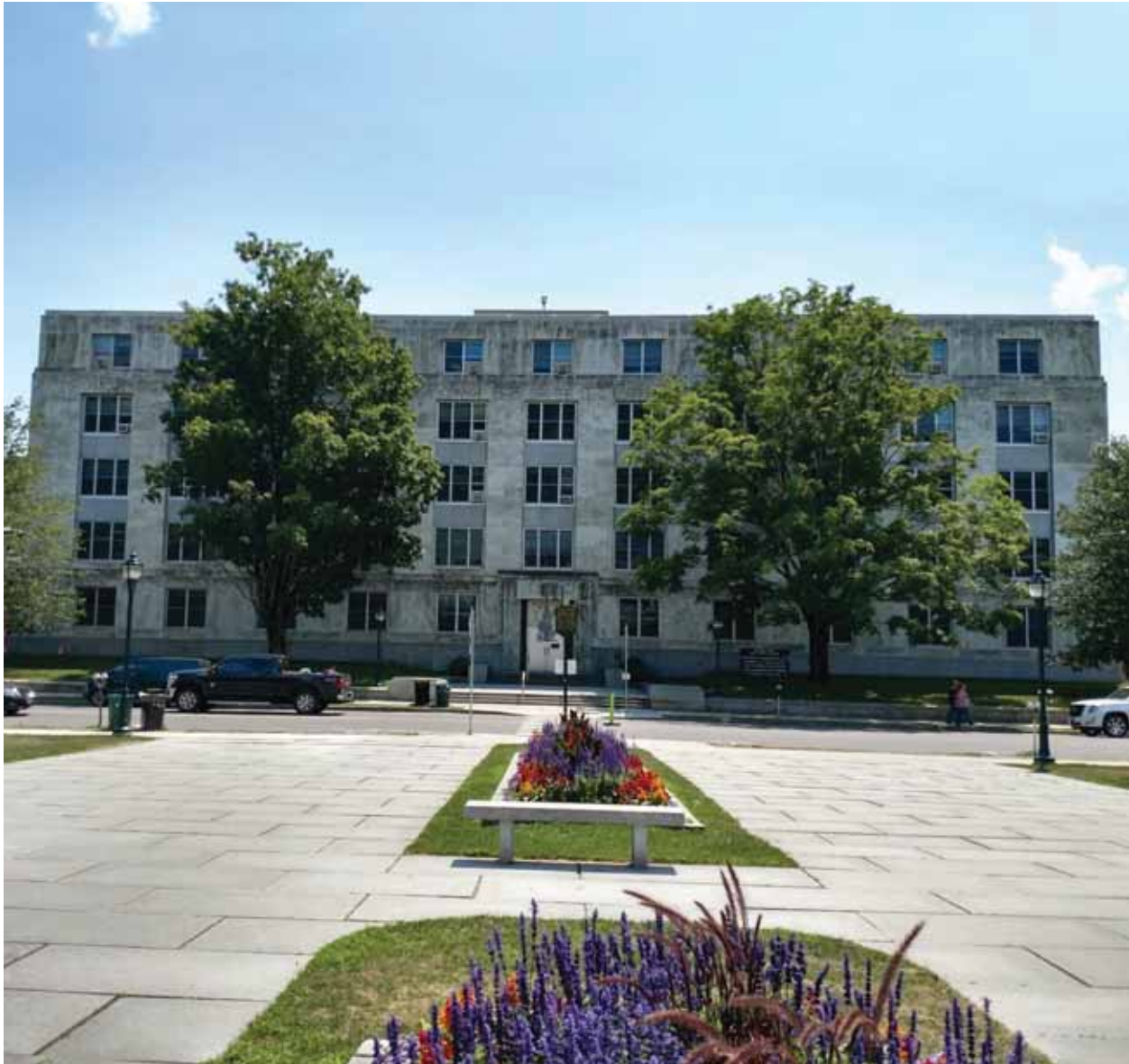
Figure 1: Front Entrance looking South (photo credit: Grenier Engineering, PC)
