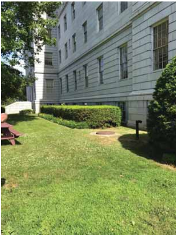
Figure 28: Basement windows (north facade), first floor at top of stairs
