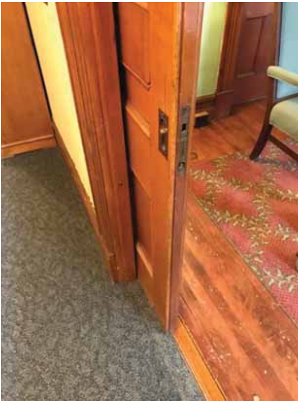
Figure 19: First floor woodwork (understood to be above predicted flood elevations)
