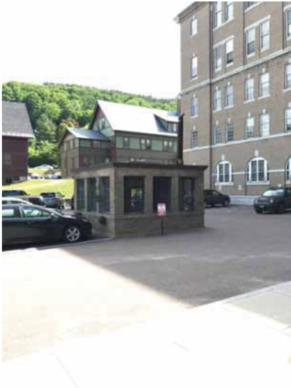
Figure 24: Roofed areaway (former ice storage tower) at the rear parking area
