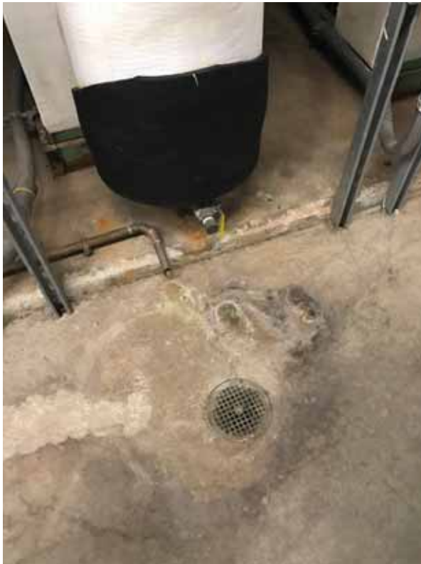
Figure 20: Sub-basement floor drain
