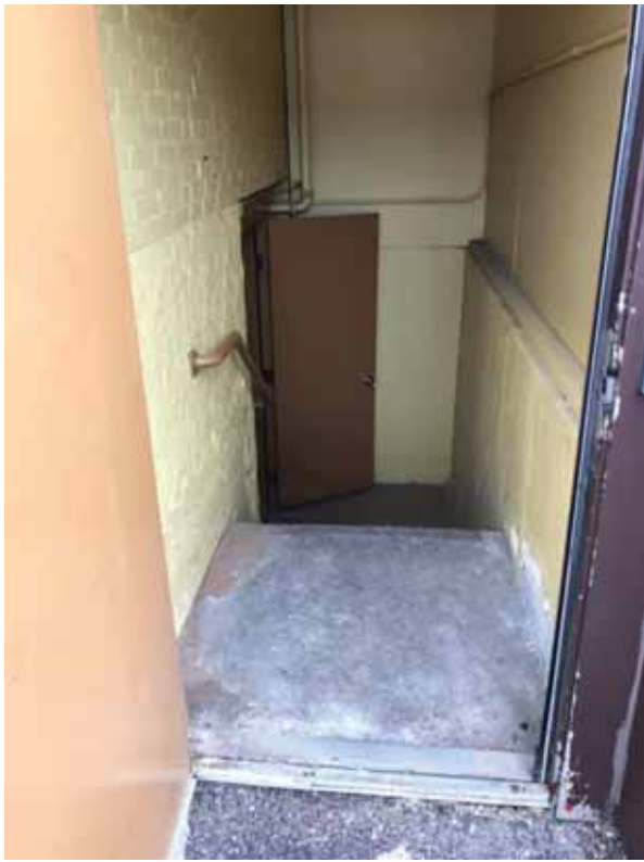
Figure 11: Basement access door open and stairs to basement
