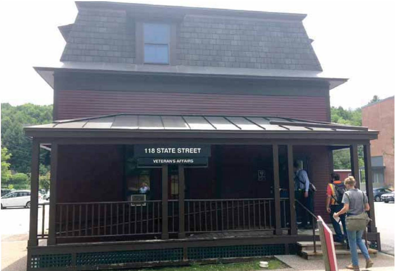
Figure 1: Front Entrance looking South (photo credit: Freeman French Freeman)
