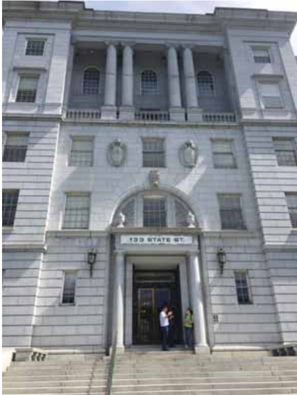
Figure 5: South façade and main entrance
