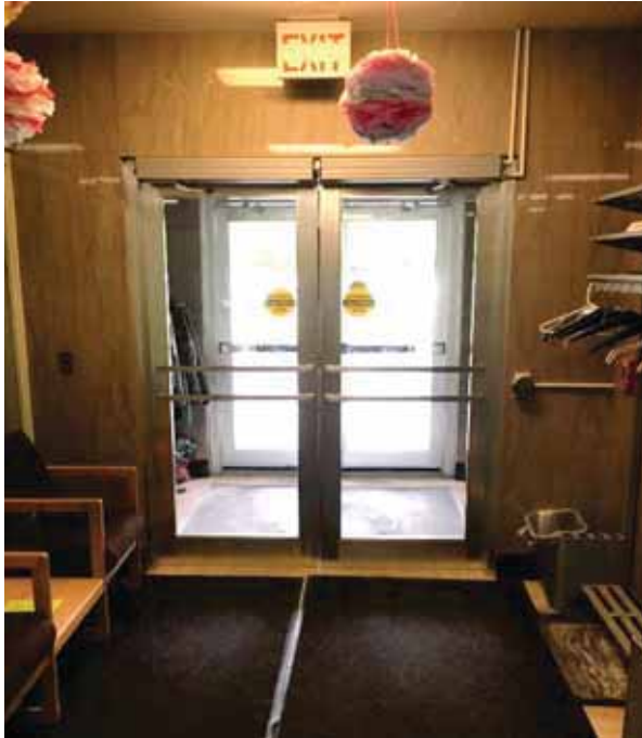
Figure 6: Basement exit door west
