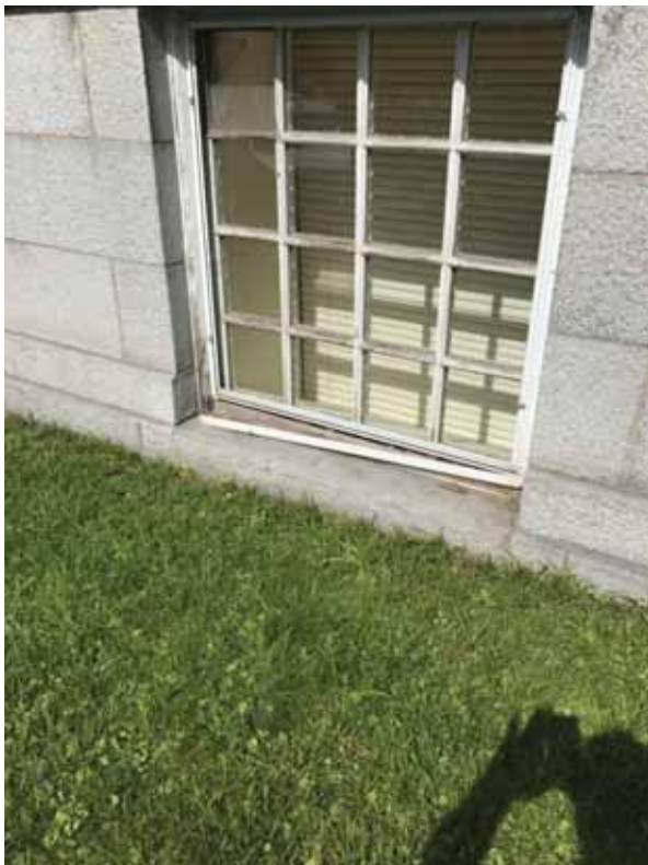
Figure 26: Basement window (typical)
