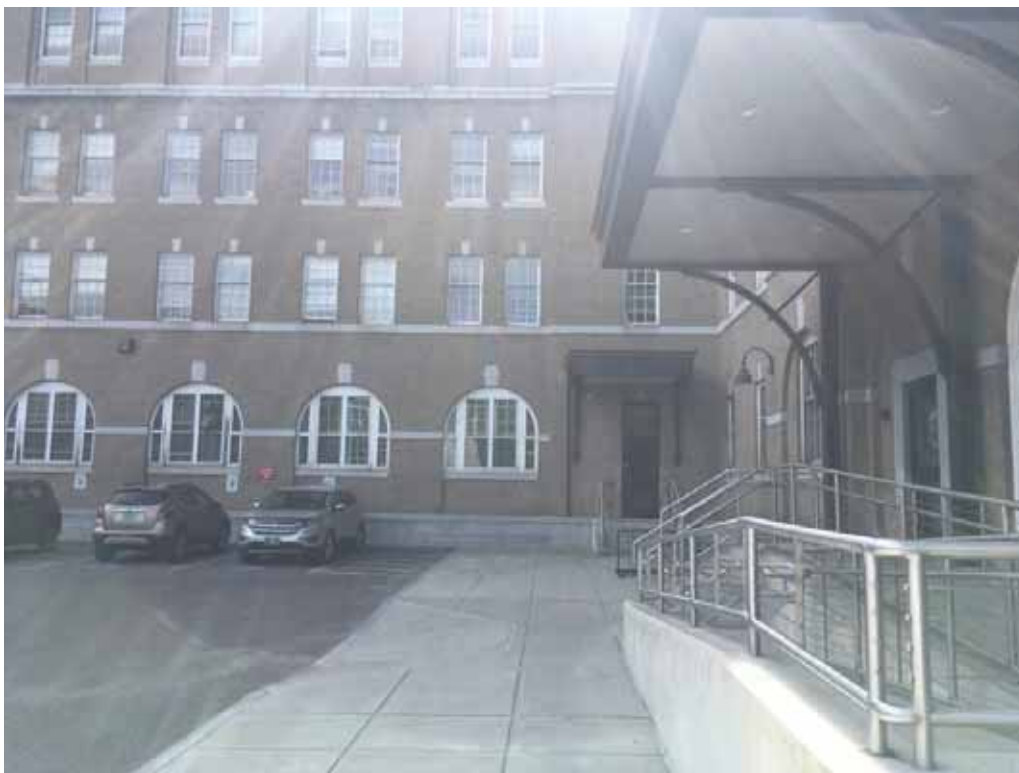
Figure 8: North and west façades
