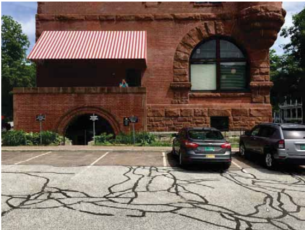
Figure 21: South façade and recessed basement entry
