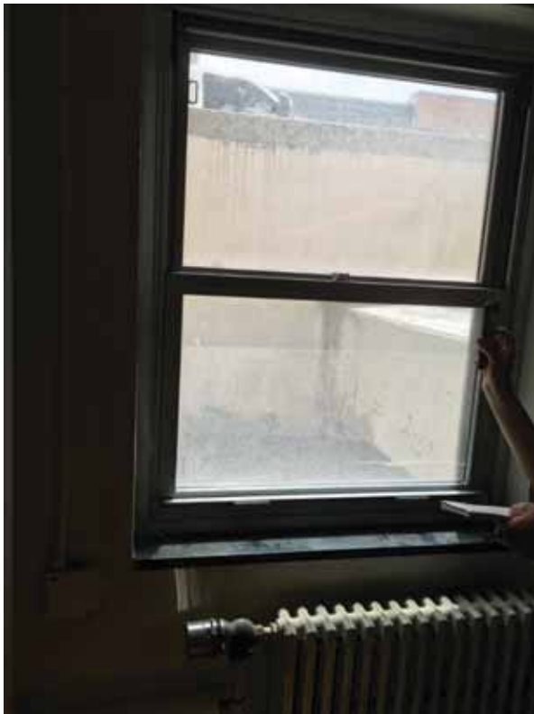
Figure 25: Basement window into areaway
