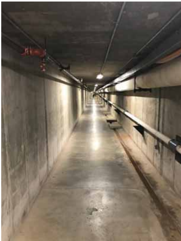
Figure 38: Basement-level tunnel across Statehouse Green
