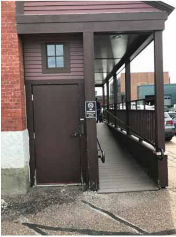
Figure 10: Basement access door
