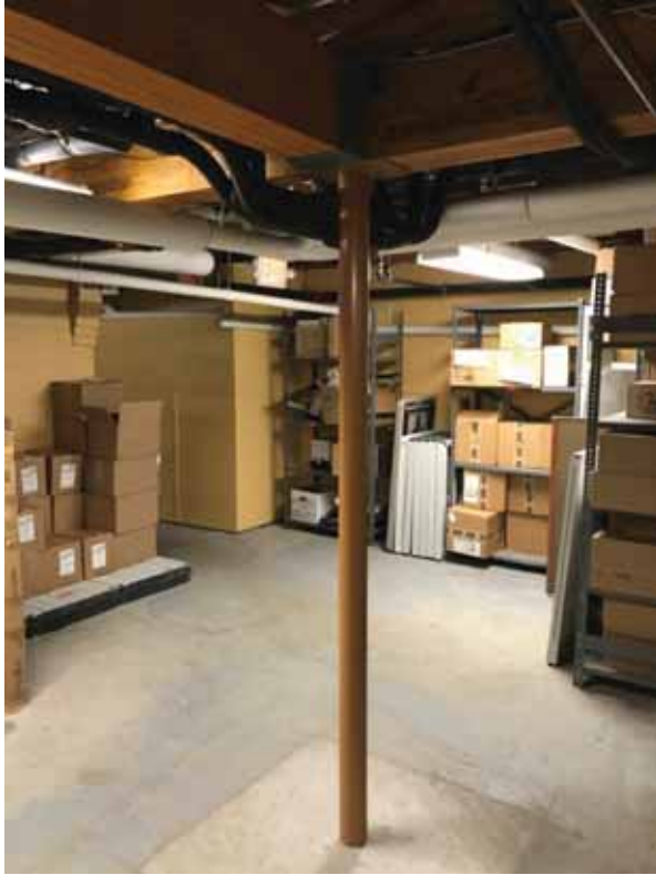
Figure 22: Basement column and stored supplies
