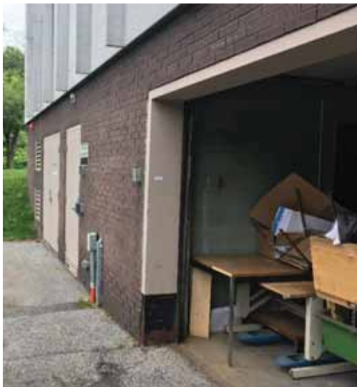
Figure 17: Openings in south façade
