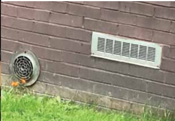
Figure 18: Vents and openings in west façade
