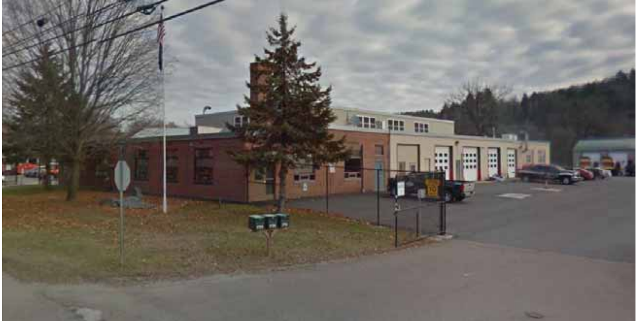
Figure 1: View of Central Garage Building looking northeast (photo credit: Google Maps)
