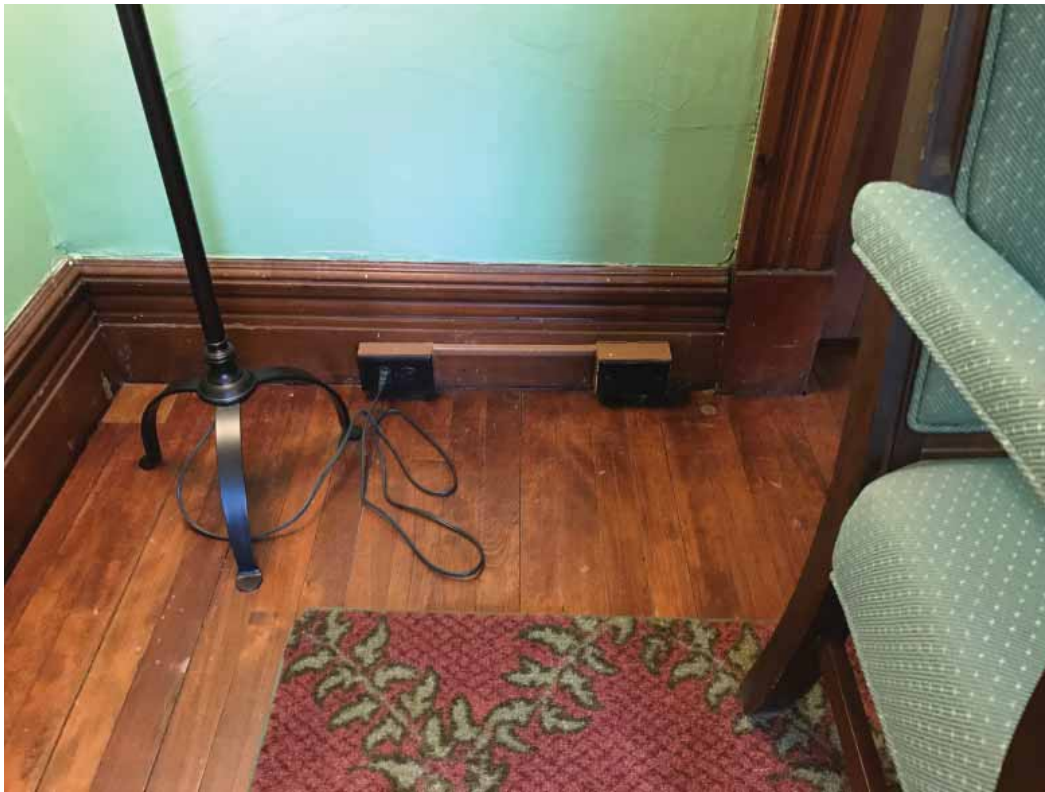
Figure 17: First floor woodwork (understood to be above predicted flood elevations)
