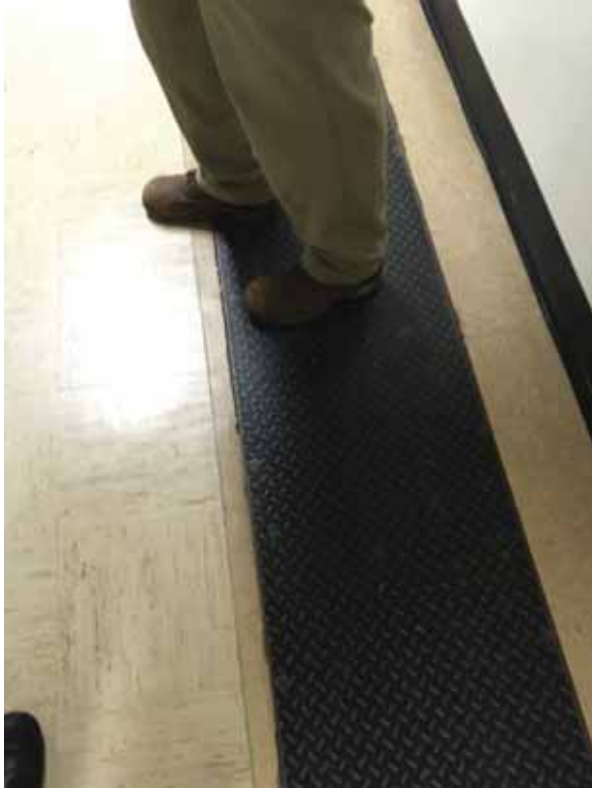
Figure 20: Basement floor trench with cover plate
