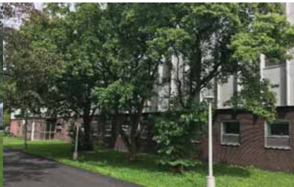
Figure 16: Building West Elevation
