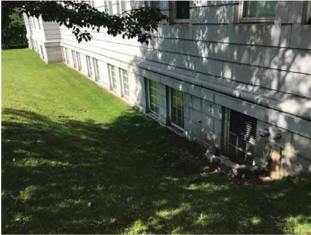
Figure 25: Basement windows at building perimeter (east façade)
