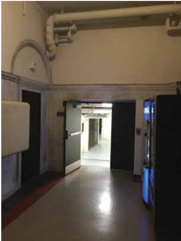
Figure 10: Basement floor looking towards tunnel and access to sub-basement
