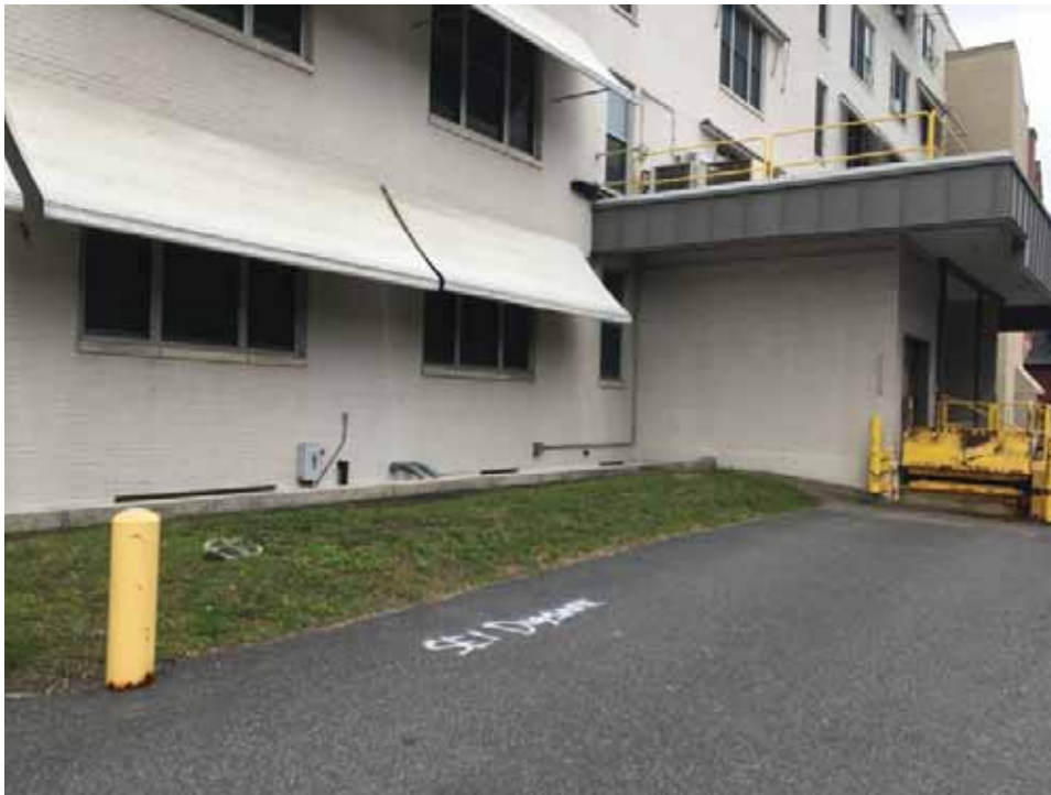
Figure 10: South areaway and loading dock
