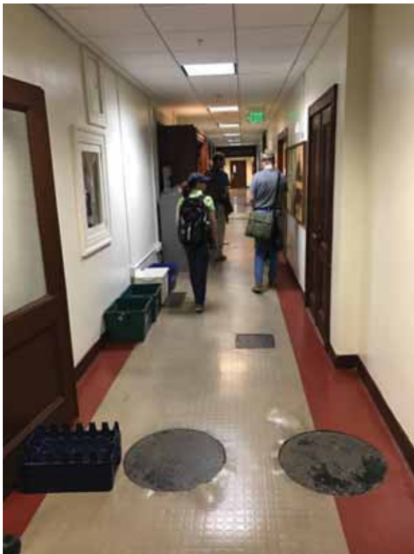
Figure 30: Basement hallway and access panels
