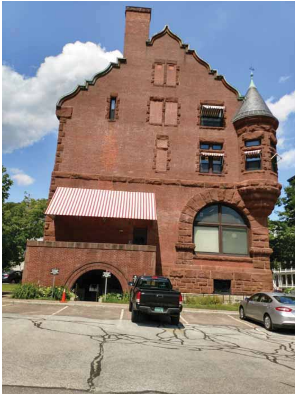
Figure 2: Rear Entrance looking North (photo credit: Grenier Engineering, PC)
