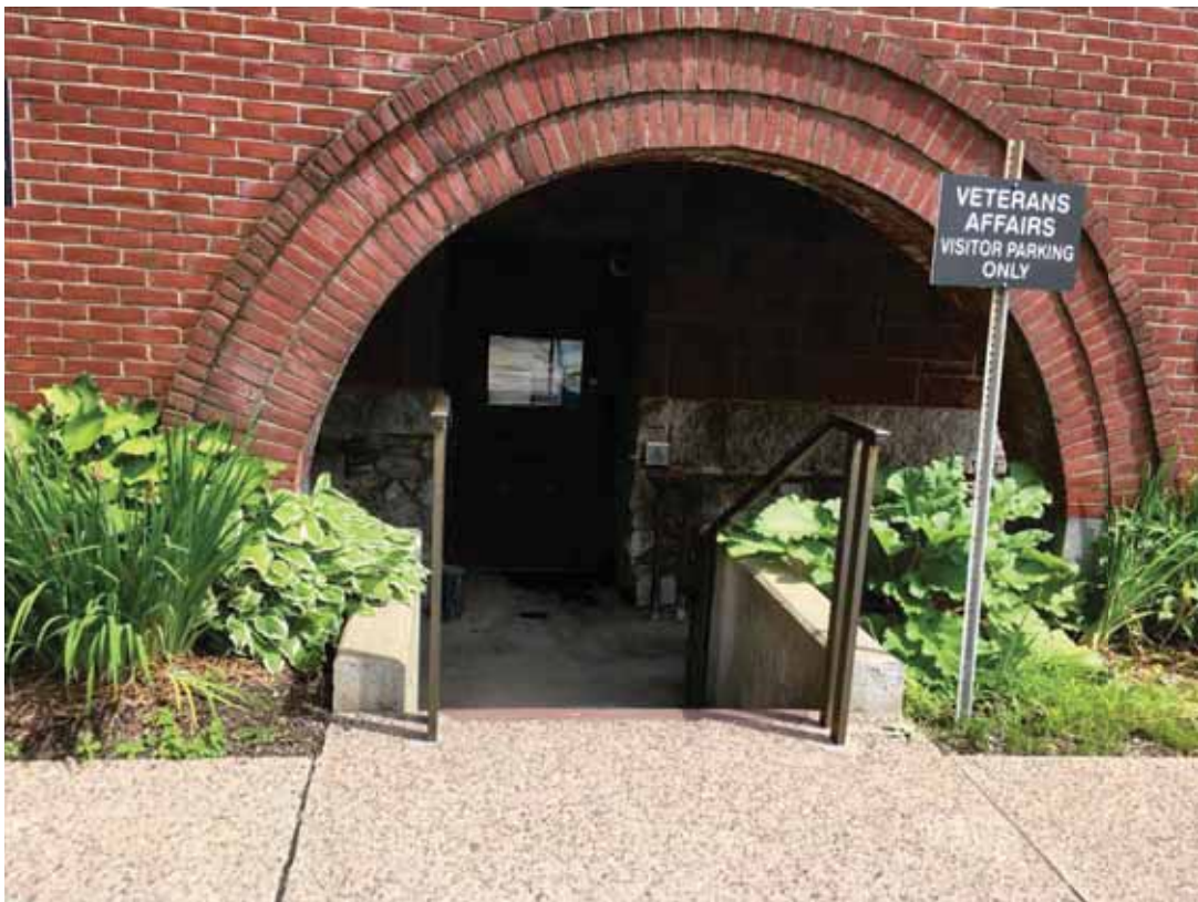
Figure 19: Basement recessed entry
