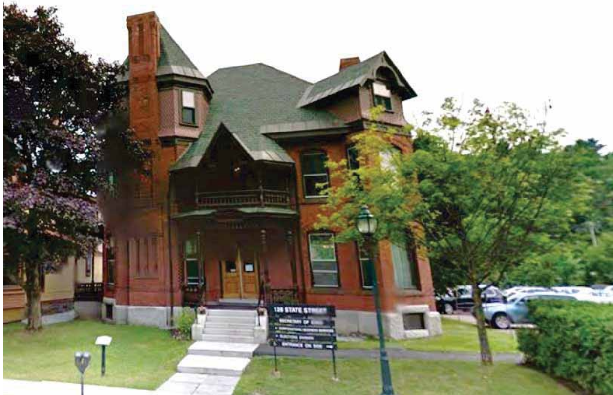
Figure 1: Front Entrance looking South (photo credit: Freeman French Freeman)
