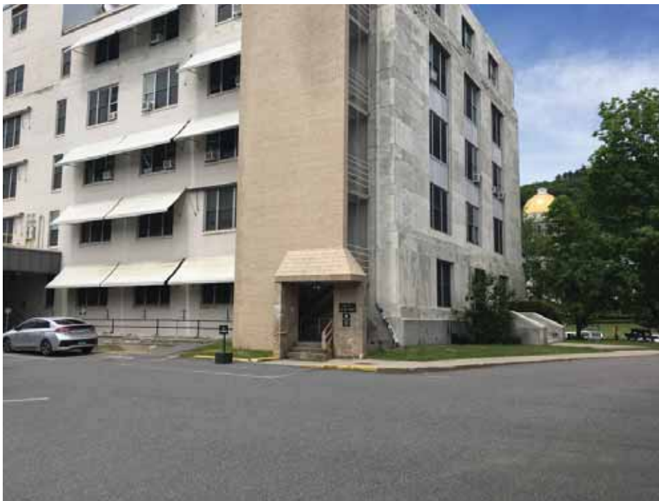
Figure 7: East and south façades
