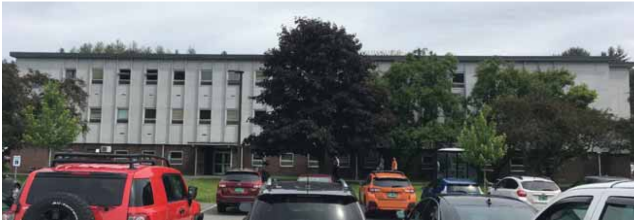
Figure 1: West Façade looking East (photo credit: Freeman French Freeman)
