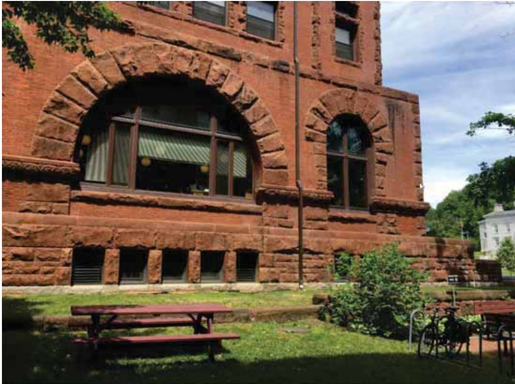
Figure 20: East façade and openings
