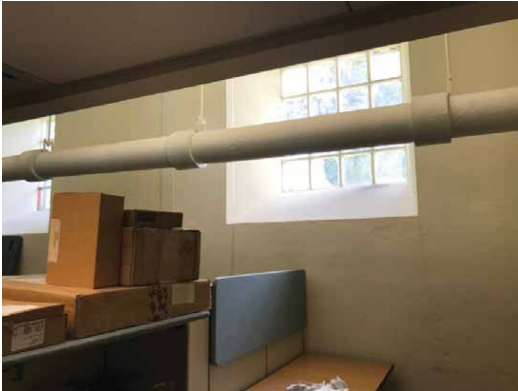
Figure 33: Basement-level office space and storage adjacent to perimeter basement windows
