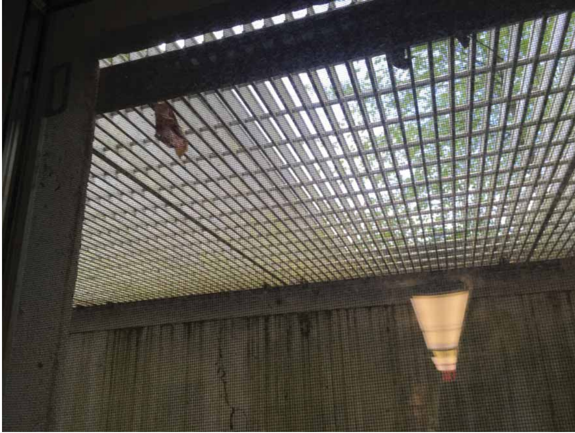
Figure 26: Areaway with grate cover
