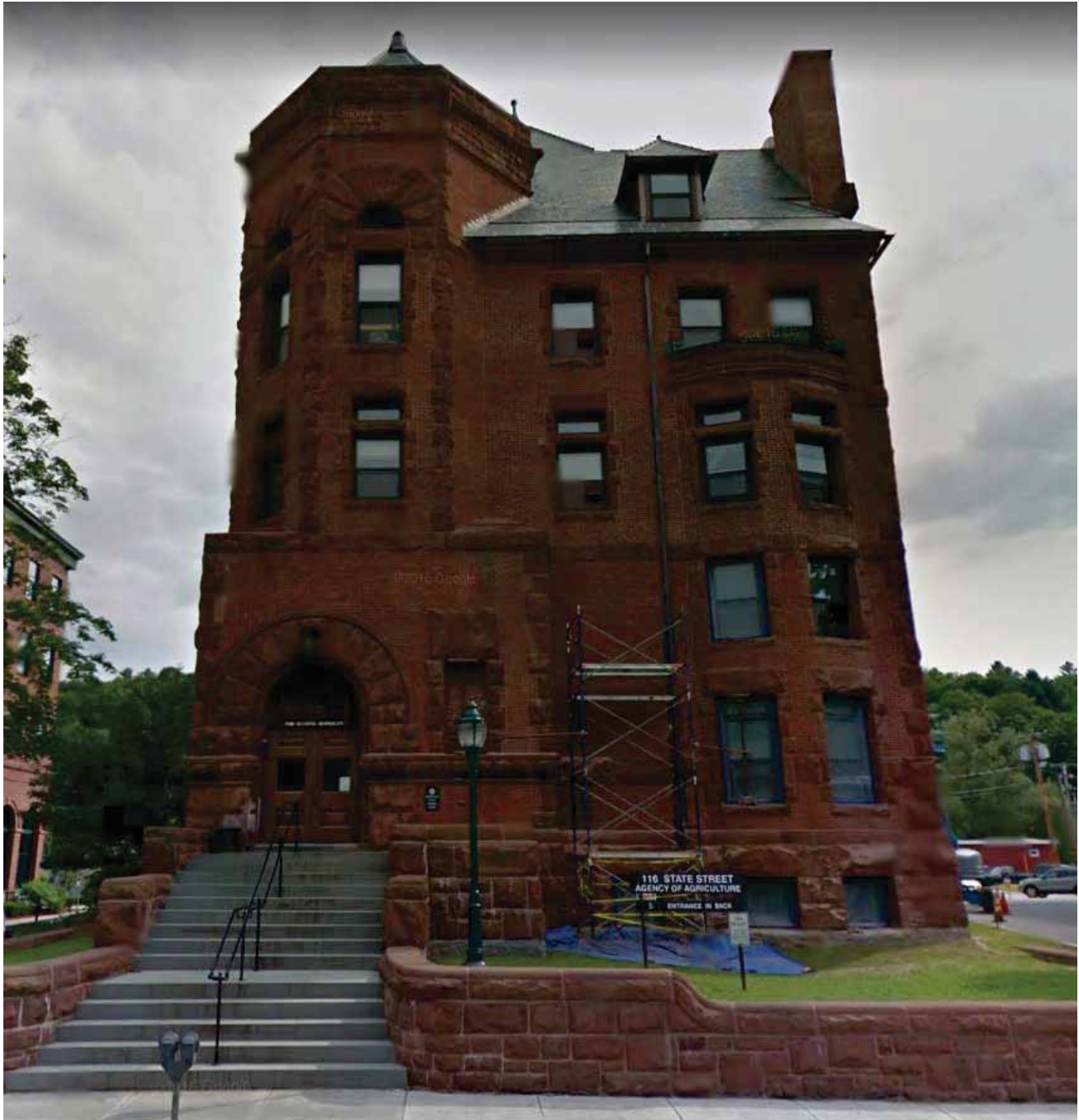
Figure 1: Front Entrance looking South (photo credit: Freeman French Freeman)
