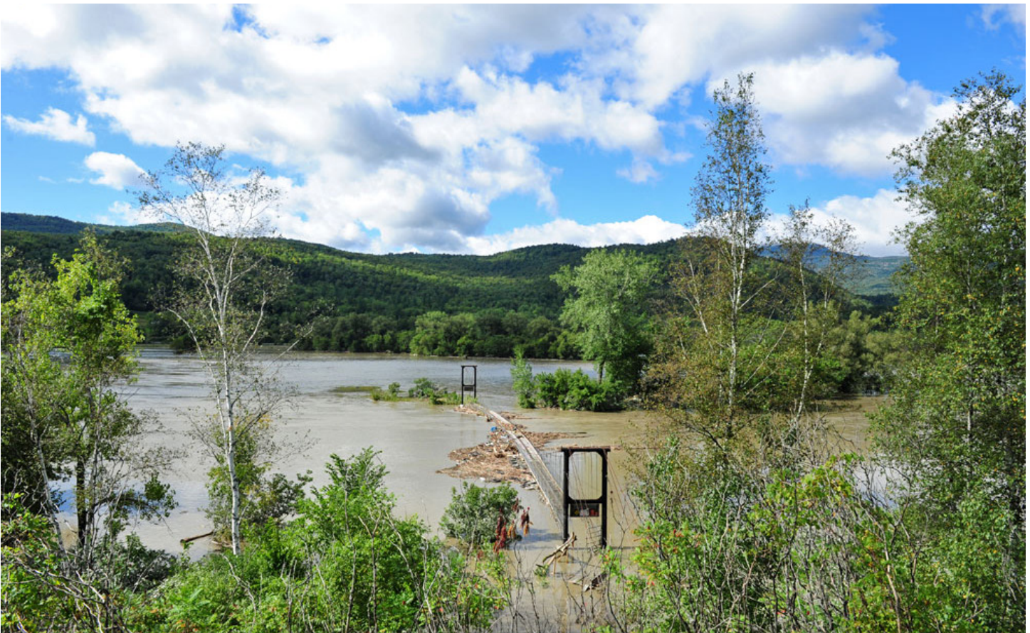
Snowmobile bridge near Waterbury, VT flexes as debris and water rush past following Tropical Storm Irene Photo Credit: www.mansfieldheliflight.com/flood
