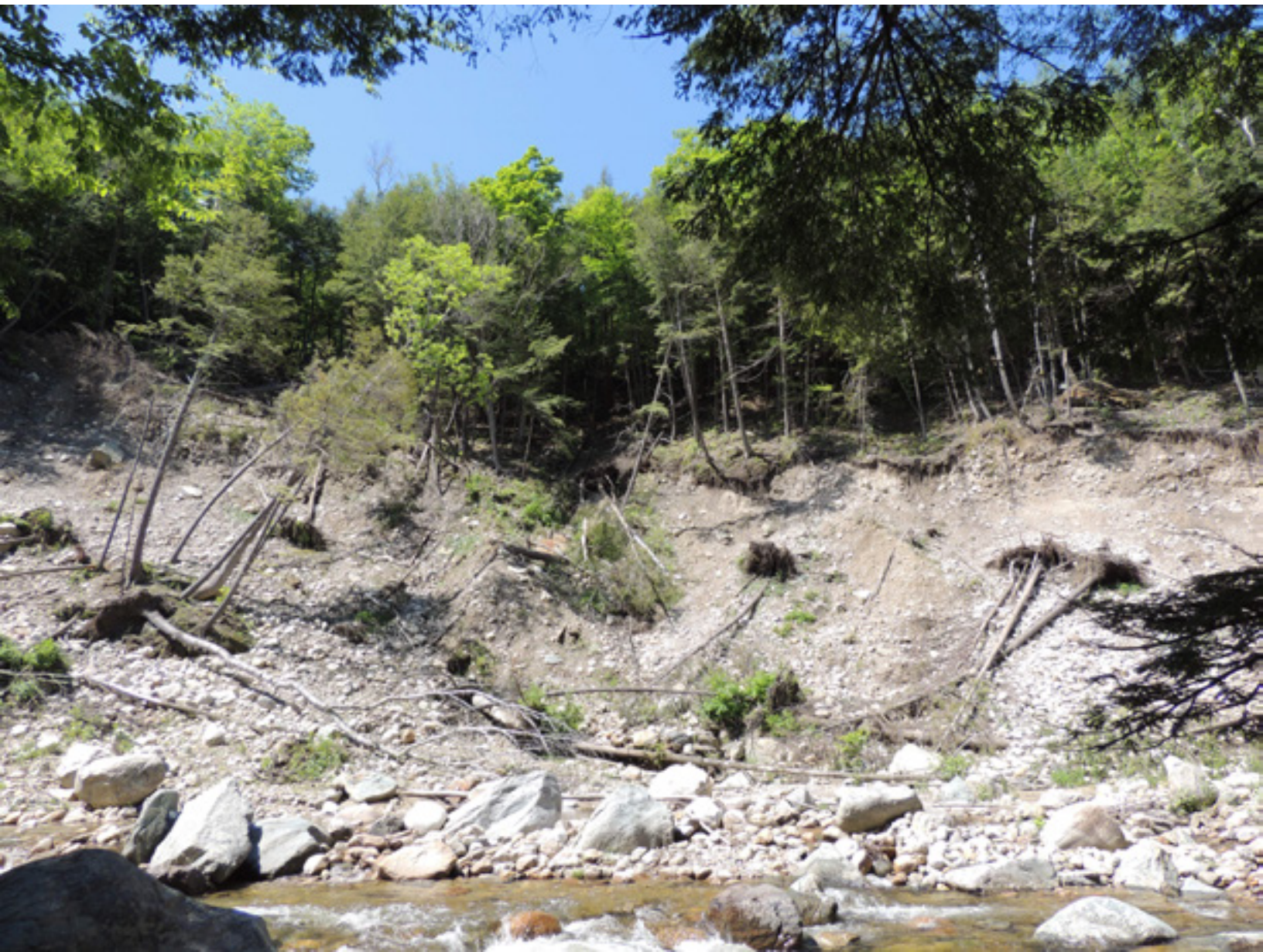
Major slope failure along the Cold River in Shrewsbury, VT. Photo Credit: Alan Shelvey
