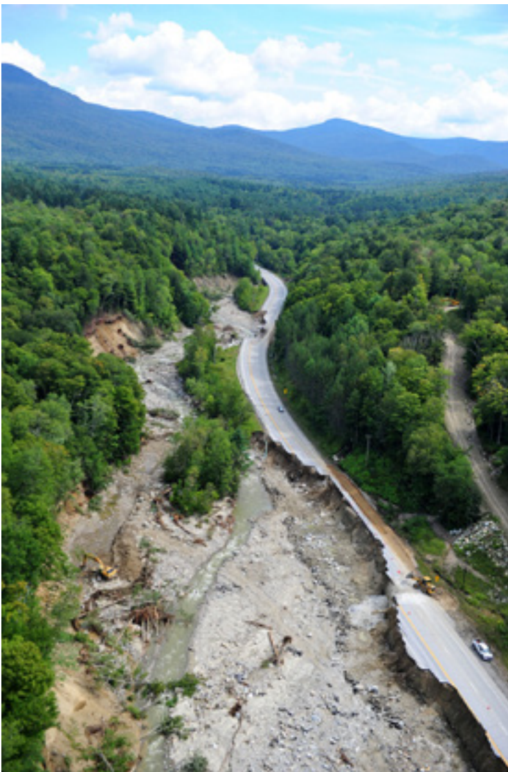
Severe damage to Vermont Route 4 in Killington, VT due to fluvial erosion during Tropical Storm Irene Photo Credit: www.mansfieldheliflight.com/flood
