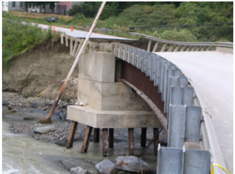
Significant scour along the Riford Brook in Braintree caused severe damage to Riford Brook Road during Tropical Storm Irene.
