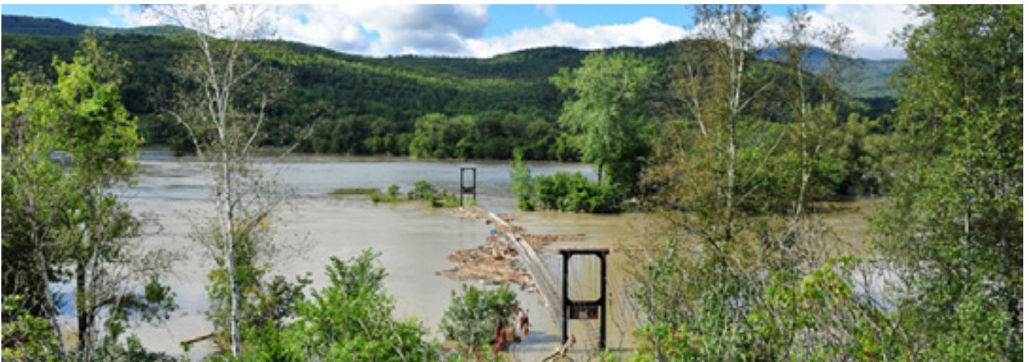
Snowmobile bridge near Waterbury, VT flexes as debris and water rush past following Tropical Storm Irene
