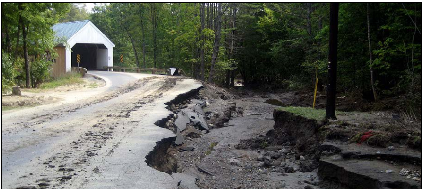
Tropical Storm Irene damage, 2011
